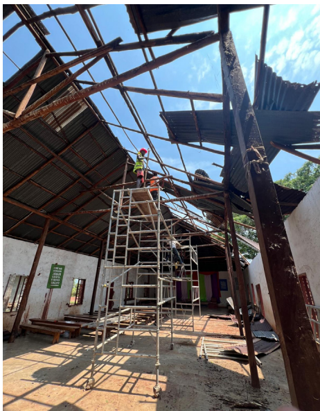
Replacing the roof sheets
