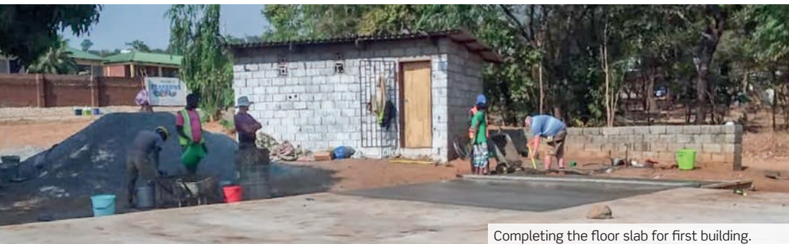
Completing the floor slab for first building.
