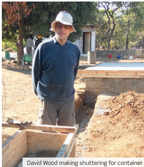
David Wood making shuttering for container
