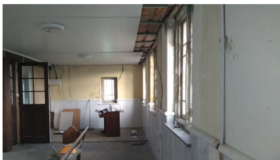
Damp walls, ceiling condensation, uneven floor
