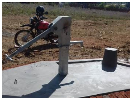
The new Afridev hand pump at Saidi will eventually be replaced with a solar electric one.
