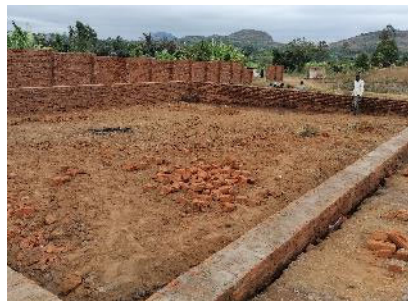
Building a base for containerised office and stores
